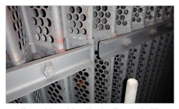
Close up of plate and channel interface, illustrating the sliding connections and range of movement
