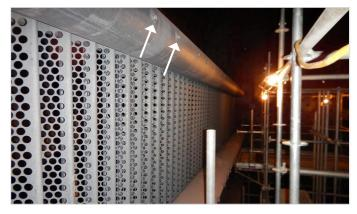
Bolts tacked to the backside of the support pipes
