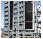
The MSG is designed for HRSGs behind gas turbines between 30 and 70 MW that allow a single gas path width. This design incorporates the ultimate in pre-fabrication and dramatically reduces the erection schedule.
