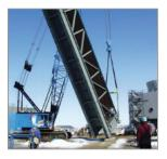
Semi-Modular Accelerated Delivery Reduced Cost Top Supported is used when shipping constraints prevent the use of the ECS design. Our SMART-Box design is highly pre-assembled; modules, casing, interconnecting piping, and some of the structural steel are all contained in each module box.
