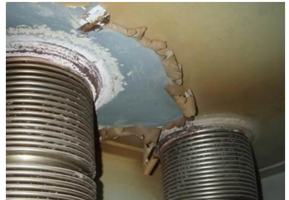
Inspection of External Penetration Hot Spot
