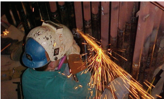
Boiler Super Heat Replacement
