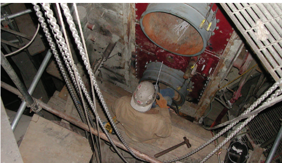
Corner Fired Burner Replacement
