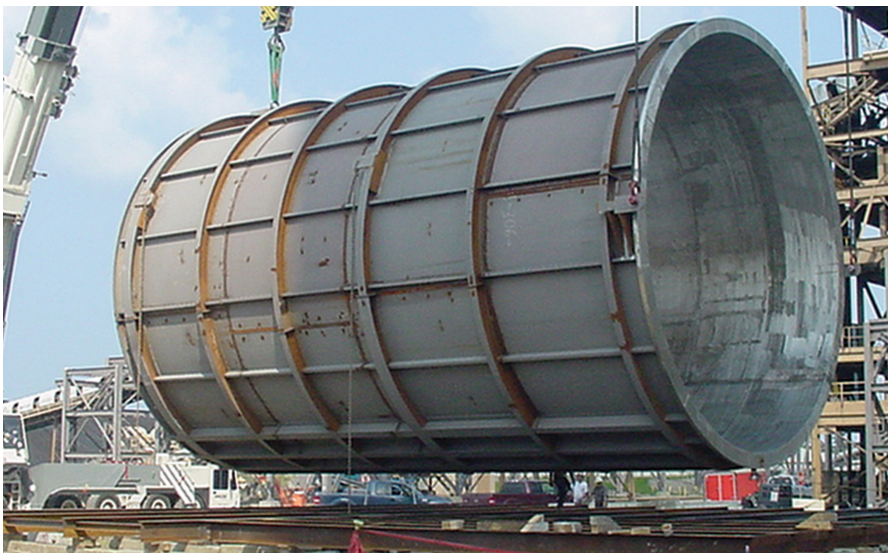
Erecting Scrubber (FGD)
