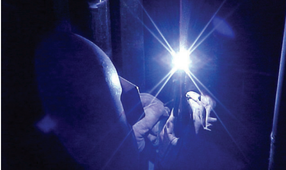
Boiler Tube Welding
